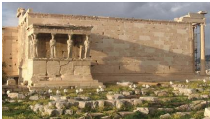
Figure 4: Erechtheion, South Wall
