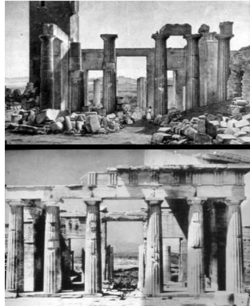
Figure 7: Propylaia east side before and after the restoration of Balanos
