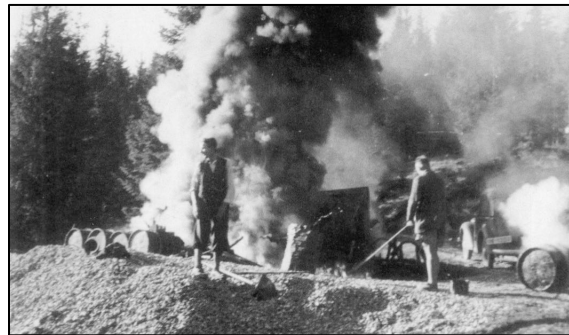
Pictured (above): Laborers working on the road
