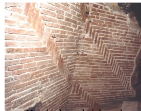
Herringbone brickwork
