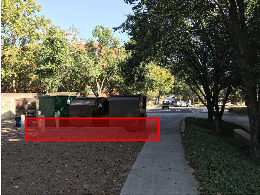
Curb and gutter removal
